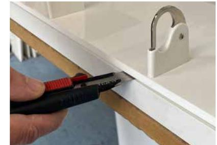
To remove the shelf, carefully cut the double-sided adhesive tape underneath using a scalpel. When replacing or reinstalling it, make sure to thoroughly clean off any remaining adhesive residue, wipe down the shelf, and apply a fresh strip of adhesive tape for secure attachment.
